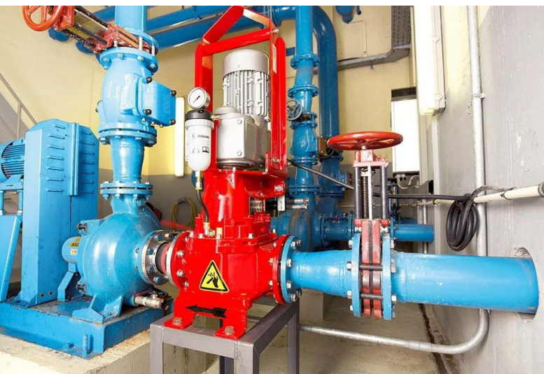
Wastewater grinder XRipper XRP136-140Q
