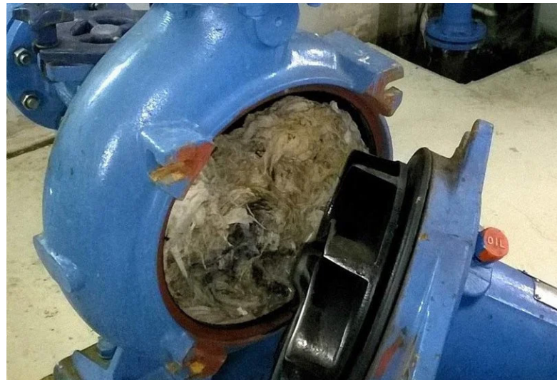
Clogged pump without XRipper
