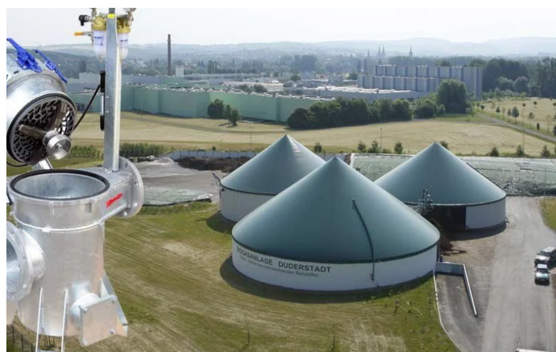
Duderstadt biogas plant
