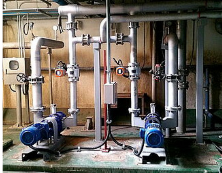
MBR filtration with rotary lobe pump: less pumps, less pipework and valves
