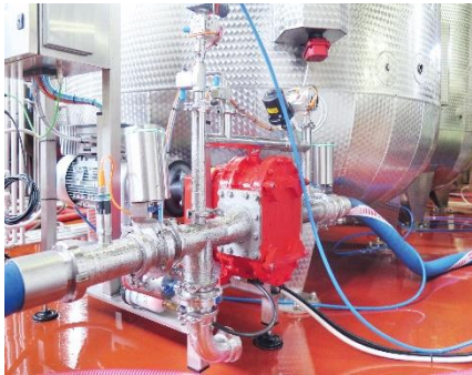
Image 3: Rotary lobe pumps from Vogelsang can also be used in fixed installations
