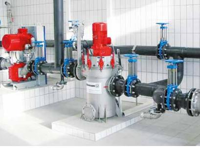
While the medium flows continuously through the RotaCut, heavy material, such as stones or metal parts, are separated out by gravity while fibers and solid matter are evenly macerate while the medium is homogenized.
