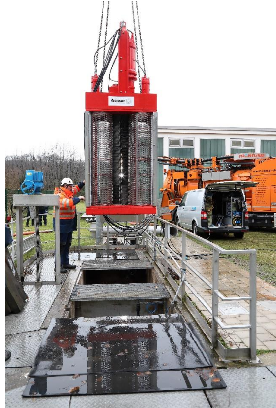
Image 2: The XRipper XRG186 during installation in the inlet of the pumping station in Witten.
